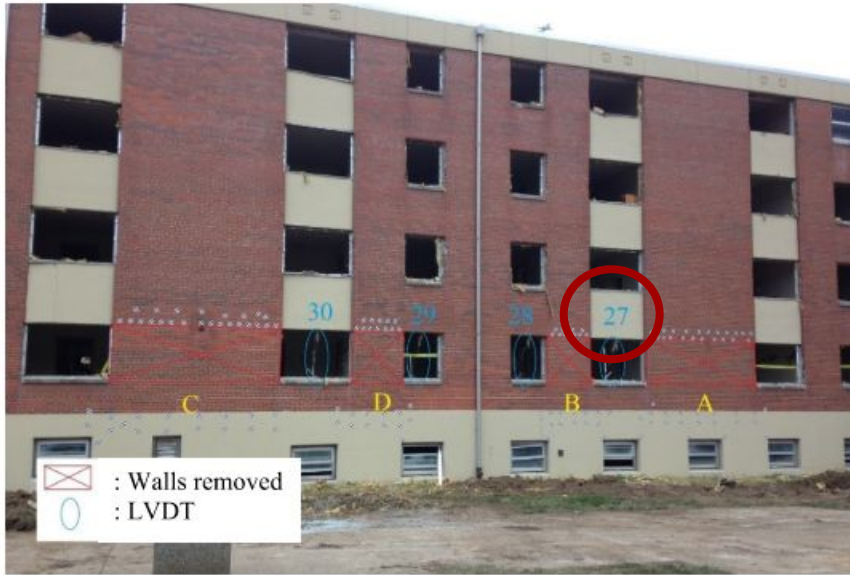
Figure 4.29: Four removed walls and LVDT numbering and locations
