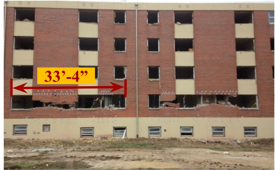
Figure 4.31: Nosker House after the removal of four walls
