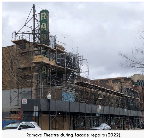
Ramova Theatre during facade repairs (2022).
